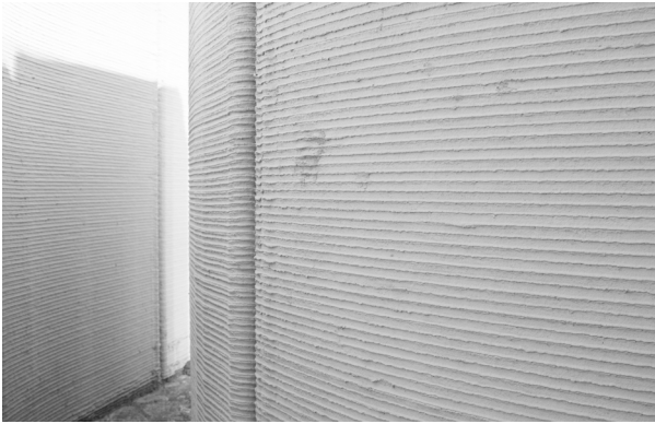
Fig. 3 - “3D Housing 05”, details of the 3D printed walls’ texture
