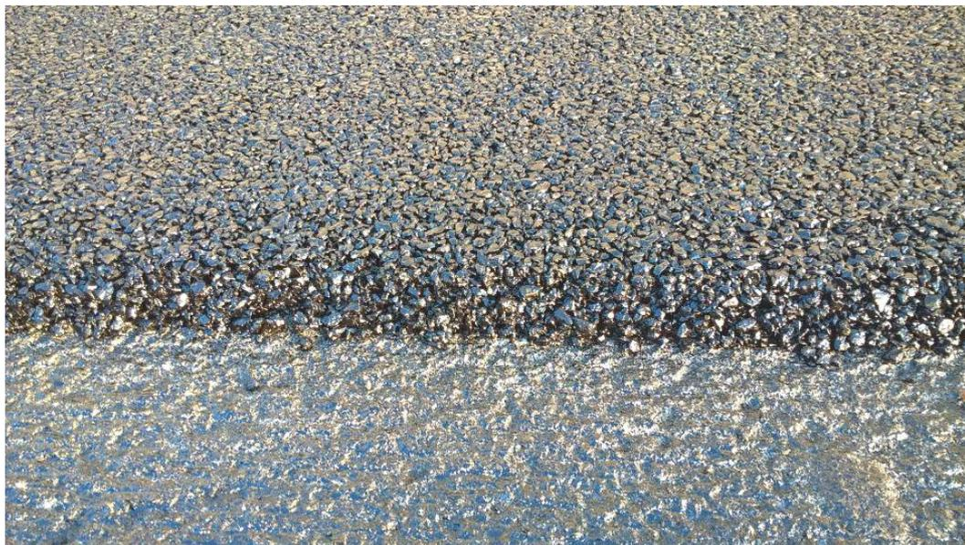
**Figura 2- Strato d'usura in asfalto open-graded.**
