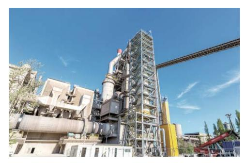
At the HeidelbergCement plant in Lixhe, Belgium, the LEILAC consortium is working on capturing CO<sub>2</sub> in its purest form, thereby reducing the ecological footprint of cement production.
